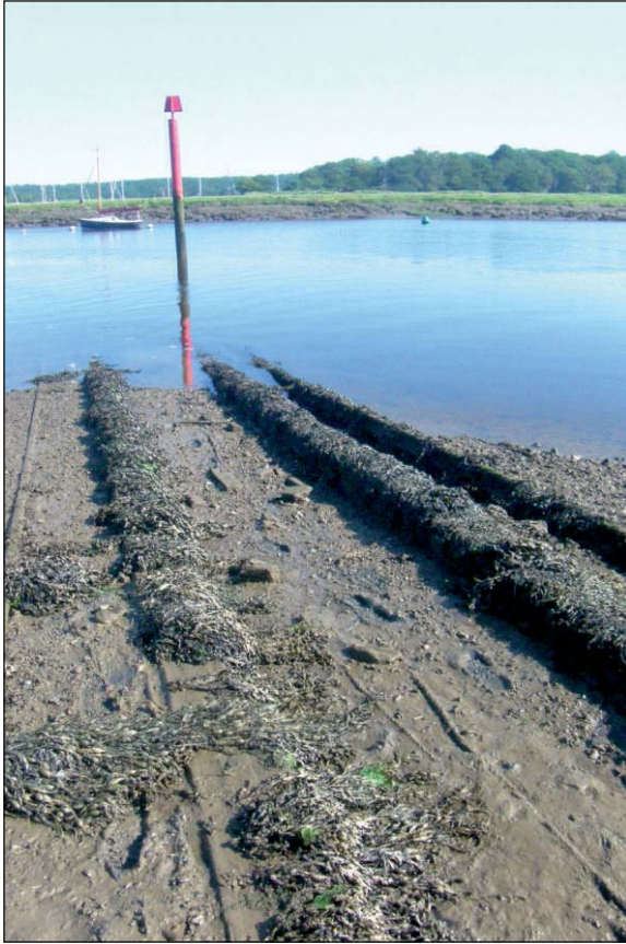
Plate 12: Lower portion of slipway, view from the south-east
