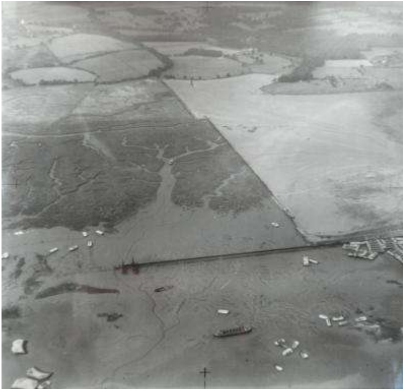
Figure 25 - EH1 RAF oblique looking west across the Test to the northern boundary of Dibden Bay in August 1947, with the breakwater laid for the next stage of the reclamation. Beetles (centre left and bottom right), concrete barges (centre right) and buffer pontoons (bottom left) are scattered throughout the area
