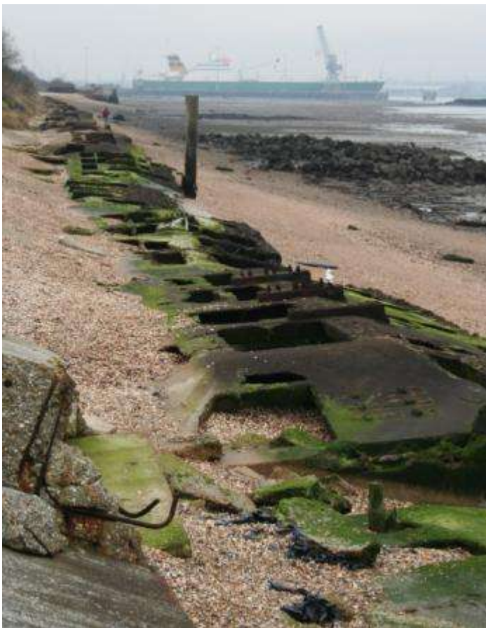
Figure 62 - Site photo looking northwest showing the predominance of dorsal algal growth at the southern end of the site, indicating that the tidal effect here is not uniform. The wooden post in Beetle no.1 and concrete remnants (possibly of a pier) can be seen in the foreground.
