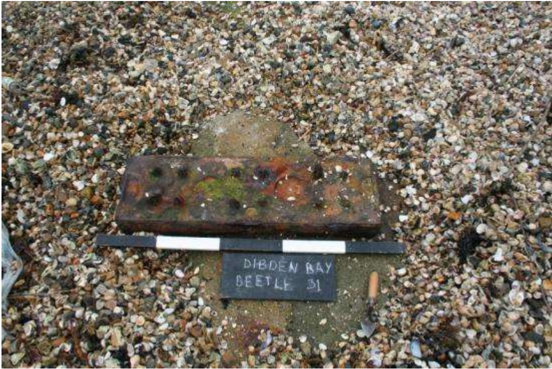
Figure 51 - Exposed dorsal coupling bracket of Beetle no.32 (not 31 as stated on slate). Trowel points to north
