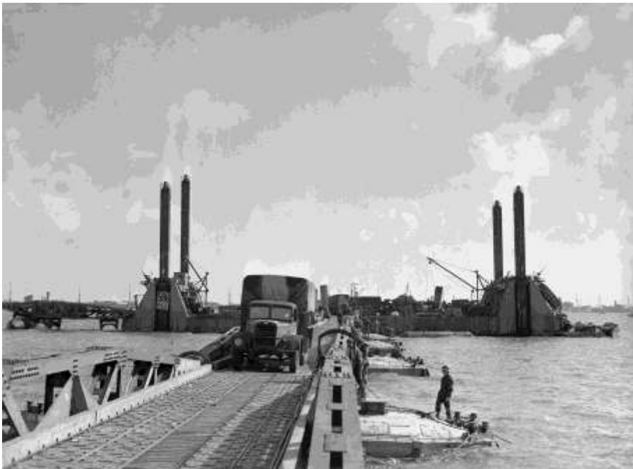
Figure 48 - Whale unit in situ in France, showing the floating roadways, the piers with hydraulic jacks and in the background, the blockships. Picture ref A-024362 IWM.
