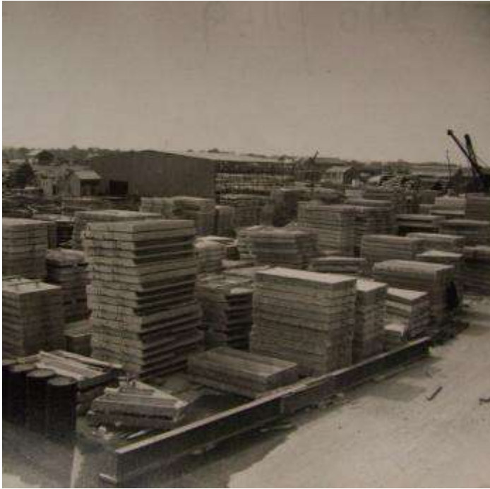
Figure 41 - Pre-fabricated concrete sections awaiting assembly at Marchwood. National Archives ref. WO 240/1159
