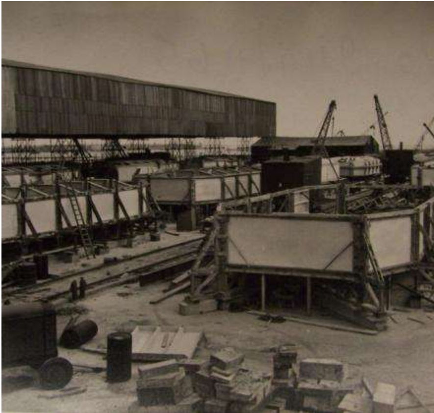
Figure 43 - Beetles being assembled in their frames ready for casting. National Archives ref. WO 240/1165
