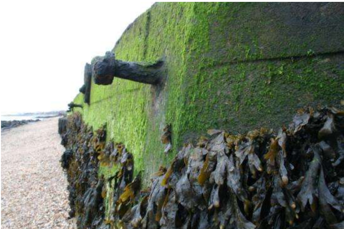
Figure 54 - Looking southeast down the line, these features were used to secure the wooden buffers and also appear in the construction photos in Section 8.2.2
