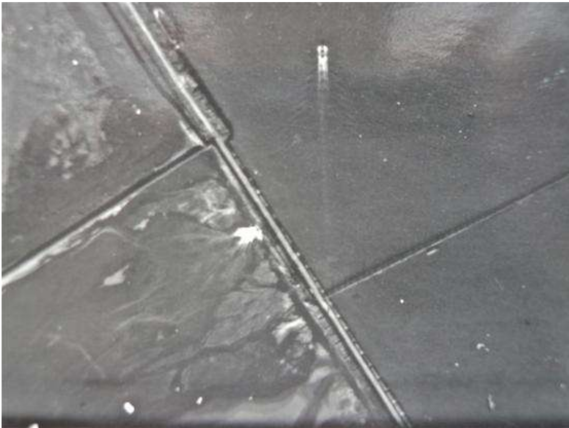
Figure 33 – Close up of EH77 showing Beetles and pier
