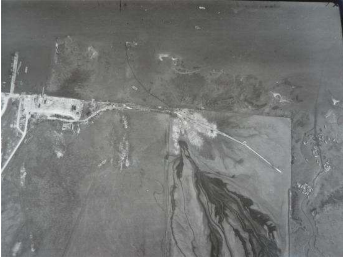
Figure 27 - EH73 April 1954. Clearance of Mulberry Harbour elements and the consolidation of Beetles in one sector to the right of the reclaim. Scale 1:9000
