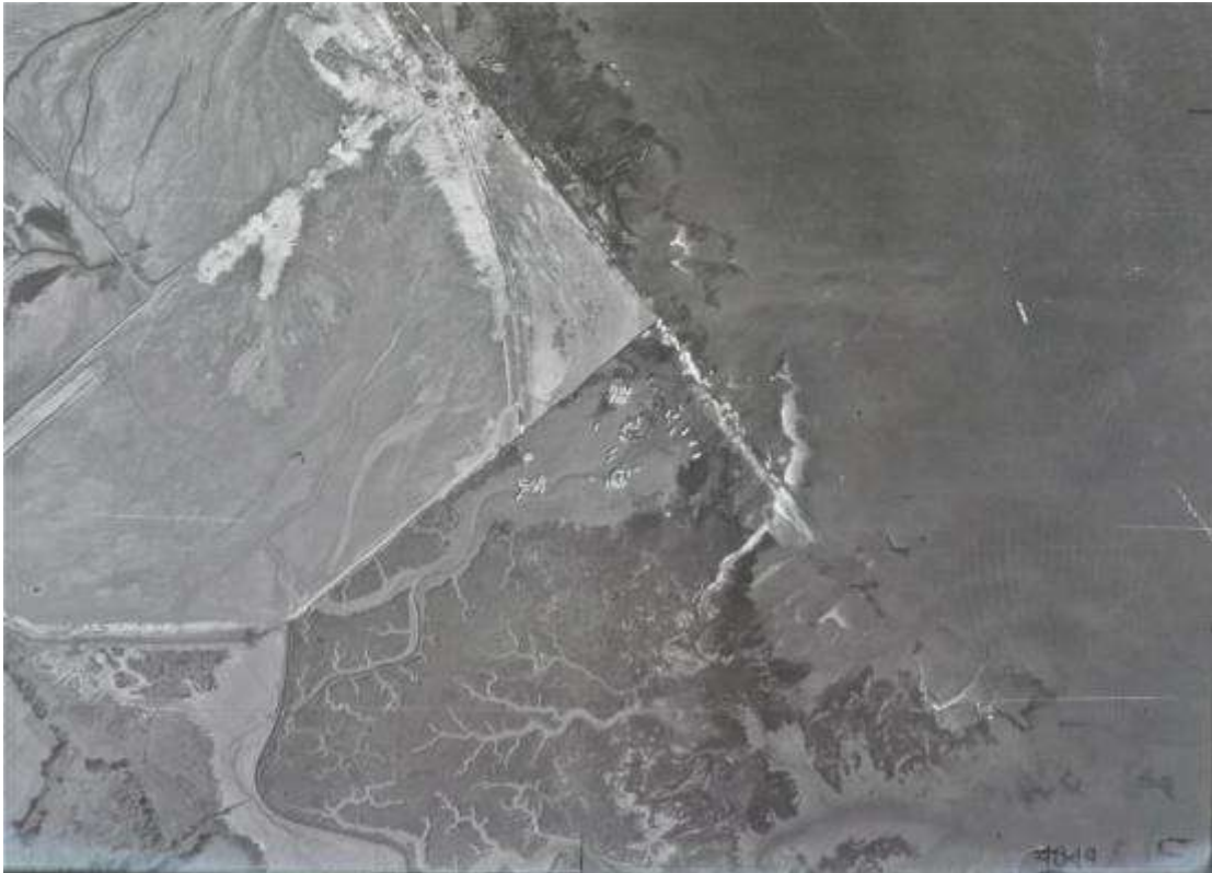
Figure 29 - EH76 July 1955. Continuation of creation of breakwater. Scale 1:10300
