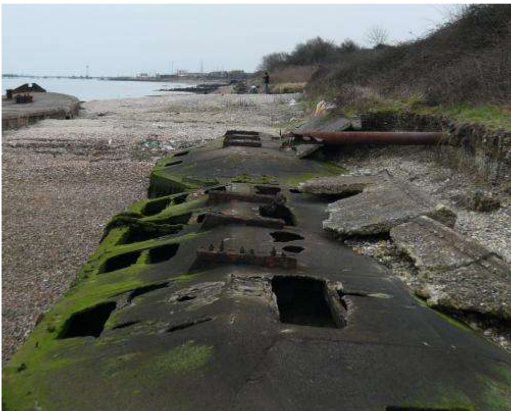
Figure 50 - Looking southeast from Section D, highlighting the shingle ridge caused by the concrete lighter to the left of picture
