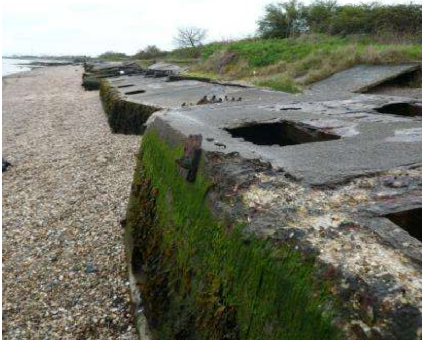
Figure 52 - Looking southeast, this photo clearly shows the alternating profiles of the Beetles
