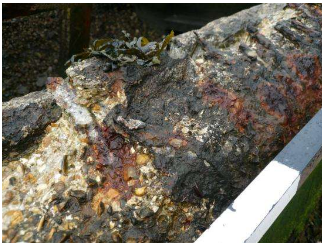
Figure 56 - Corrosion stains
