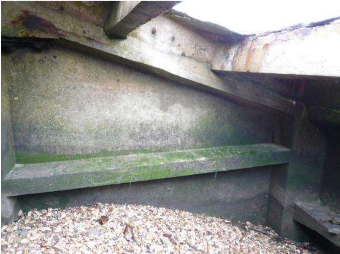
Figure 57 - Interior of Beetle showing the durability of the internal bulwarks used to create the watertight compartments
