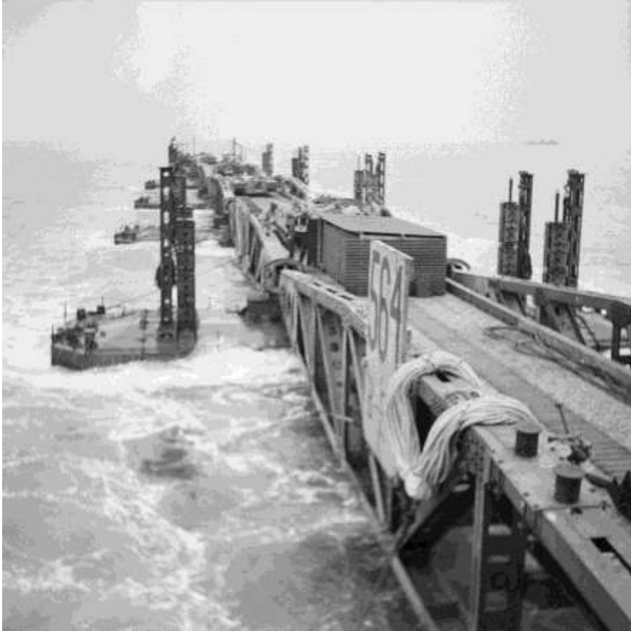
Figure 47 - Whale unit being towed to France. Note the hydraulic jacks on the Beetles indicating that these are made of steel not concrete. Picture ref B-005689 IWM
