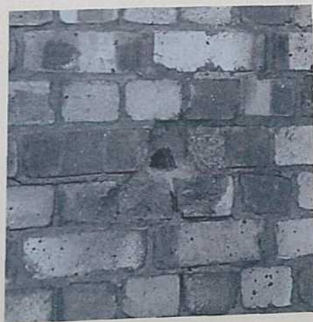
(a) Front of wall showing entry crater.
